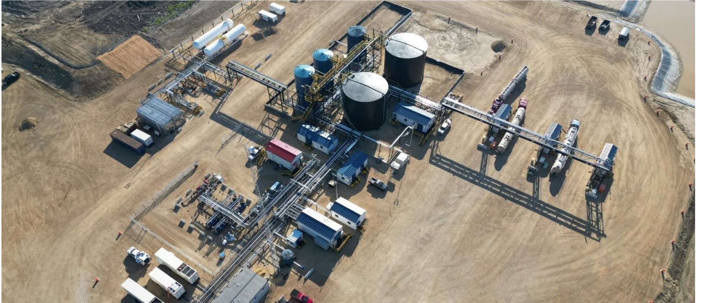
Nipisi Terminal in Northern Alberta
